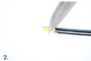
2. Use the knife and cut of the isolation from one of the conductor
