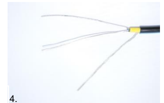
4. Carefully strip back the conductive core to expose the wire conductors. Ensure that they are not damaged
