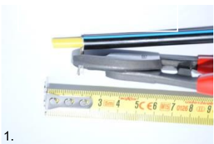
1. Strip back the outer jacket 20 mm and cut the earth wire at the end of the outer jacket
